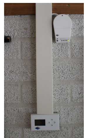
Regeling decentrale binnenunit (onder) CO 2 -indicator (boven) in klaslokaal
